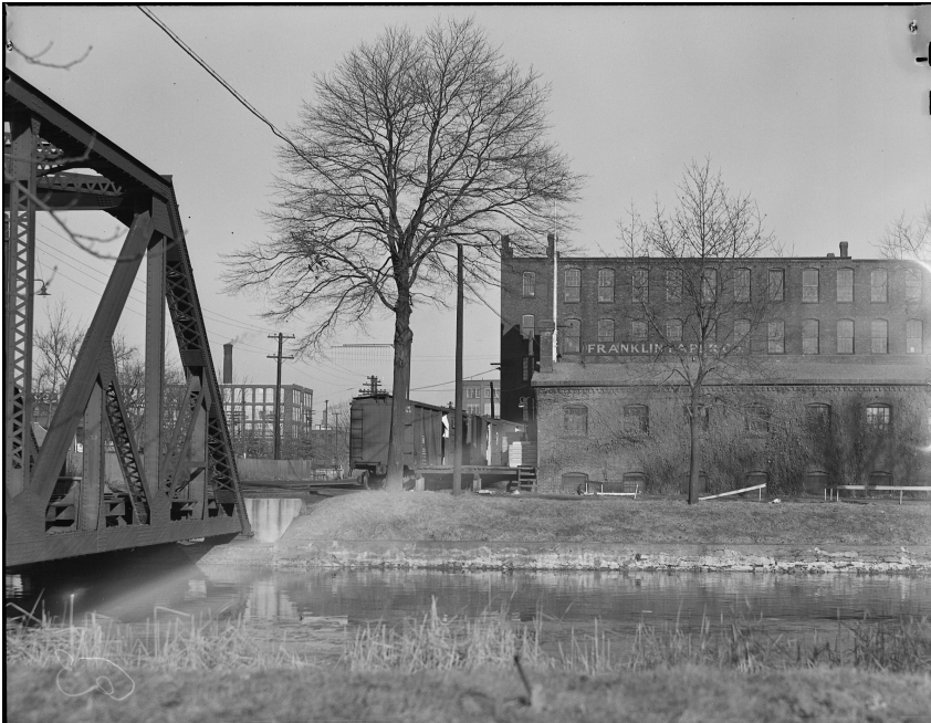
A PAPER MILL ON A HOLYOKE CANAL, 1936-37
