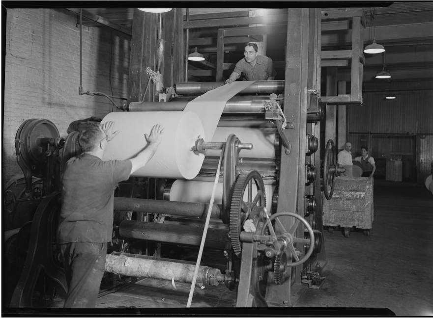
A SUPER-CALENDER IN A HOLYOKE PAPER MILL, 1936-37
